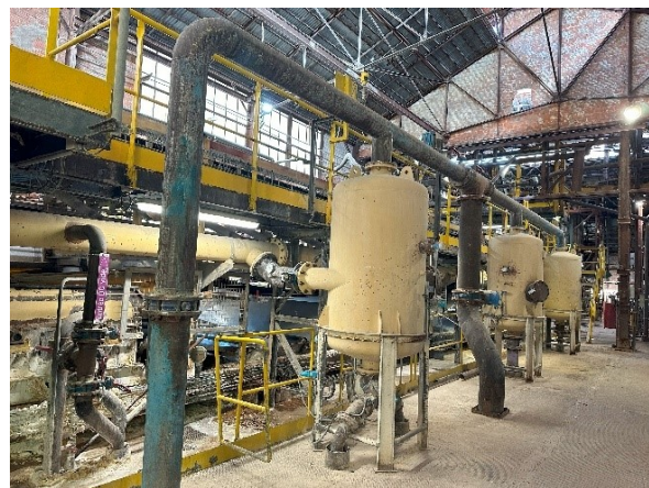
Figure 4. Left: how the new vacuum header would arrive between BA105 and BA104; Right: New Vacuum Supply header as installed with BA104 with new flange for additional liquid level indicator.
