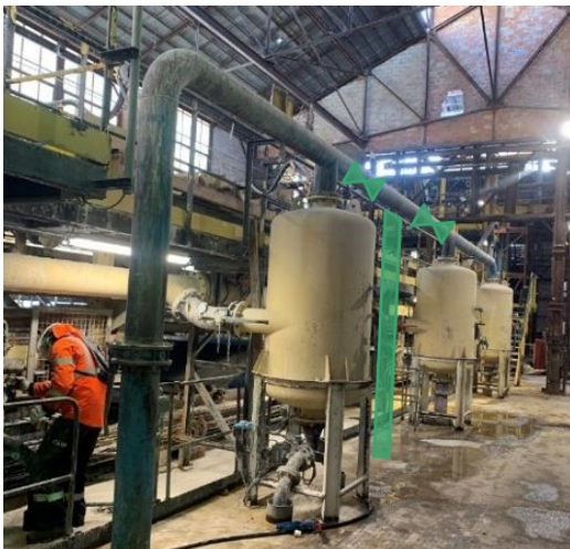
Figure 4. Left: how the new vacuum header would arrive between BA105 and BA104; Right: New Vacuum Supply header as installed with BA104 with new flange for additional liquid level indicator.
